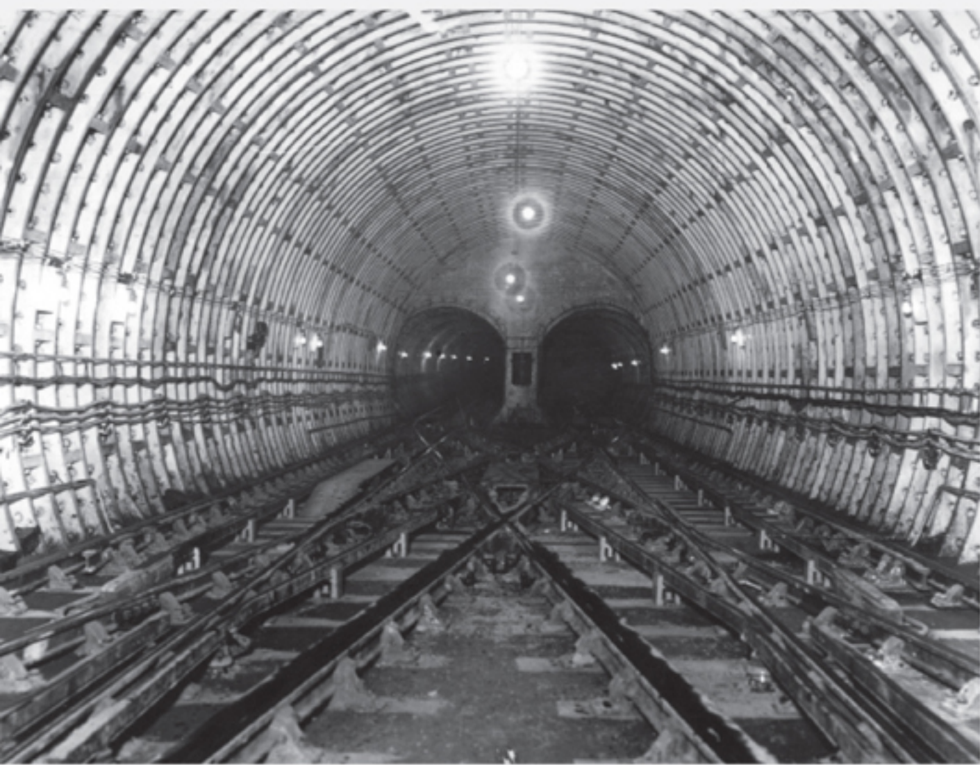
FIG 1 View of the west crossover of the London Underground's Central London Railway extension at Liverpool Street Station, 100 yards from the station, 1912.
